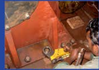
HTW-8D BEING USED ON BEML ROPE HOVEL DRUM FOUNDATION BOLTS.
