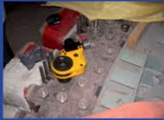
HTW-5S BEING USED FOR TIGHTENING CORE STUD BOLTS IN BHEL SITE.
