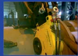
HTW-75S BEING USED AT JSL-STEEL PLANT ORISSA FOR TIGHTENING COUPLING BOLTS
